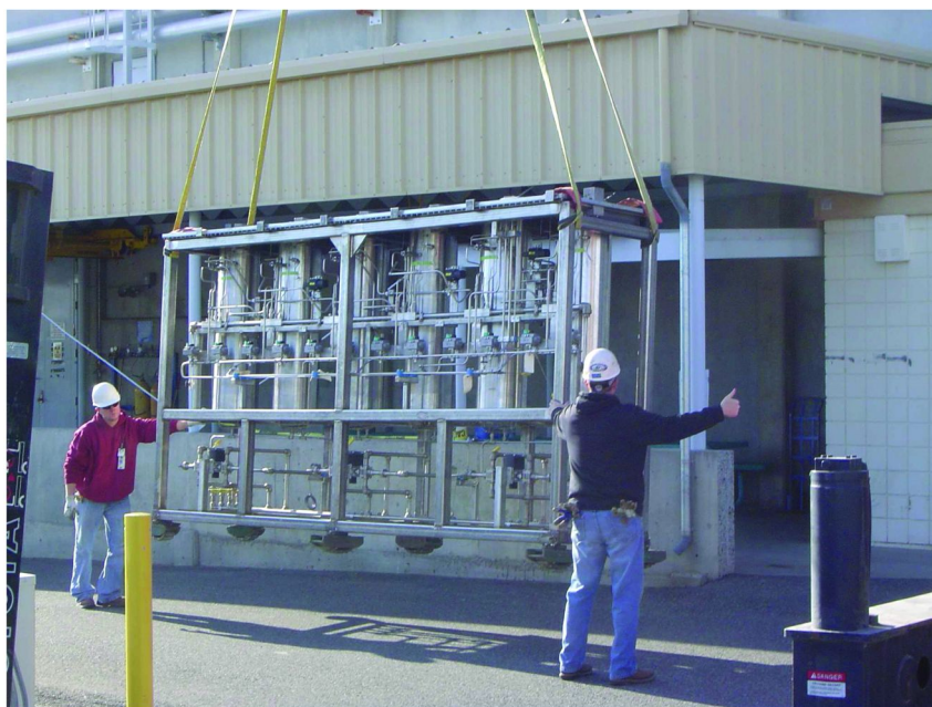
Figure 9. Extraction Module Delivery
